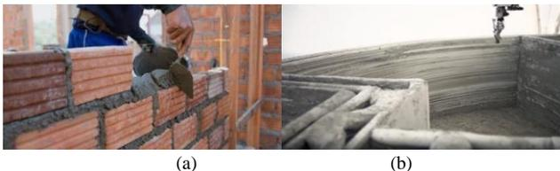
Fig. 2. (a) traditional construction (b) 3D printed construction [https://medium.com/@Nik\\_chen/what-is-construction-3d-printing](https://medium.com/@Nik_chen/what-is-construction-3d-printing) (date 29/1/2018 11:05pm)
